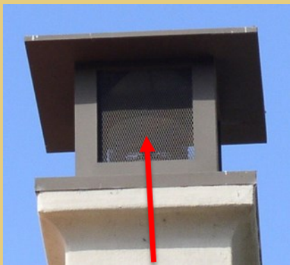
Appropriate spark arrester
