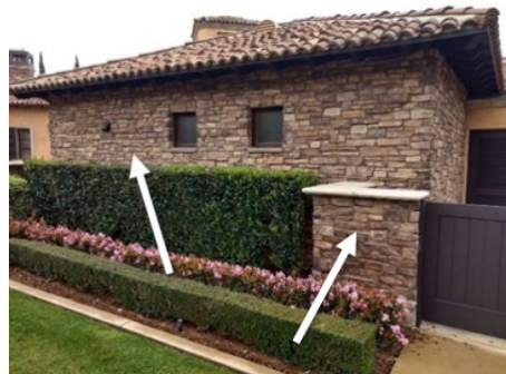
Non-combustible wall and siding
