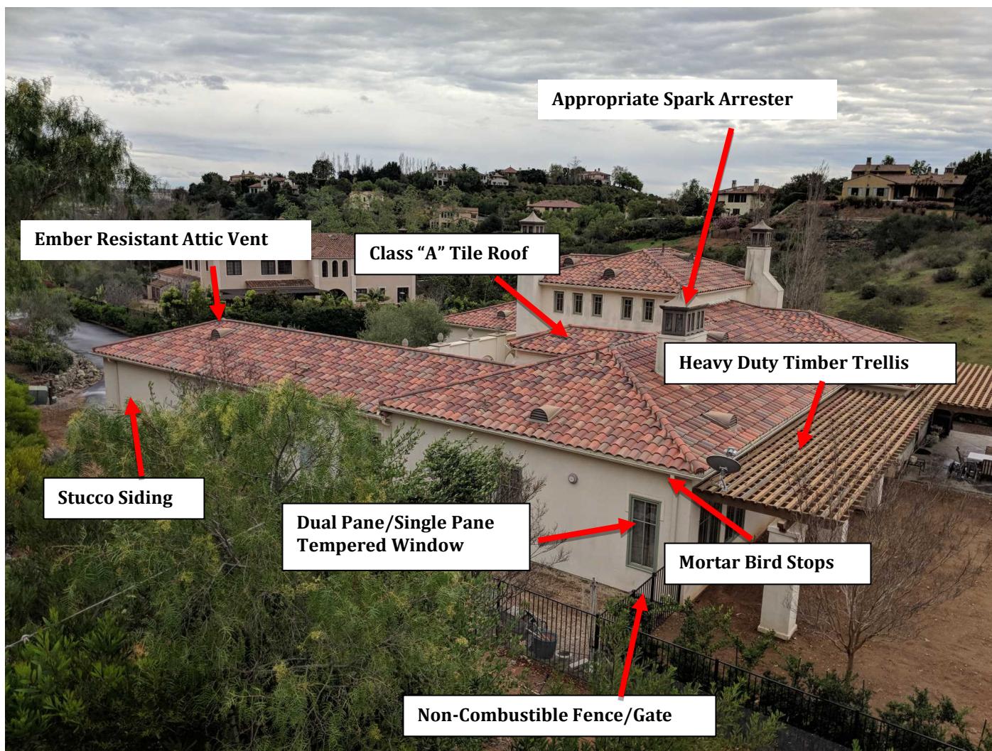
Appropriate spark arrester
