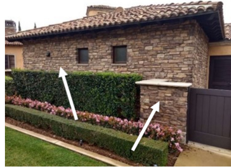
Non-combustible wall and siding
